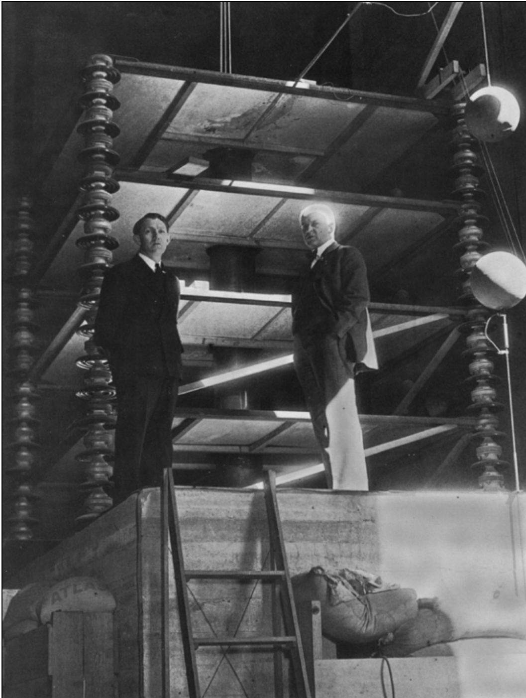
Fig. 6. Charles C. Lauritsen and Robert A. Millikan stand atop the one-million-volt X-ray tube, developed and built at Caltech by Lauritsen and colleagues in 1928. In 1931, Millikan persuaded the Detroit cornflake magnate W. K. Kellogg to finance a new laboratory to house research. Photo by Wide World Photos, Caltech Archives.
